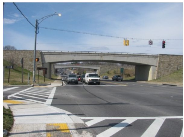
Figure 6-32. Baltimore-Washington Parkway Bridge
